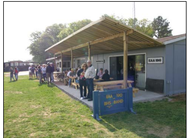
New Patio cover and concrete deck built by EAA Chapter 190
